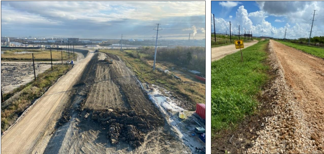
Contract PAV01 during and after construction
