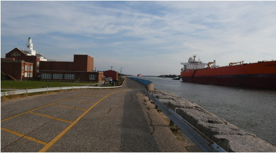
Existing Floodwall in Port Arthur
