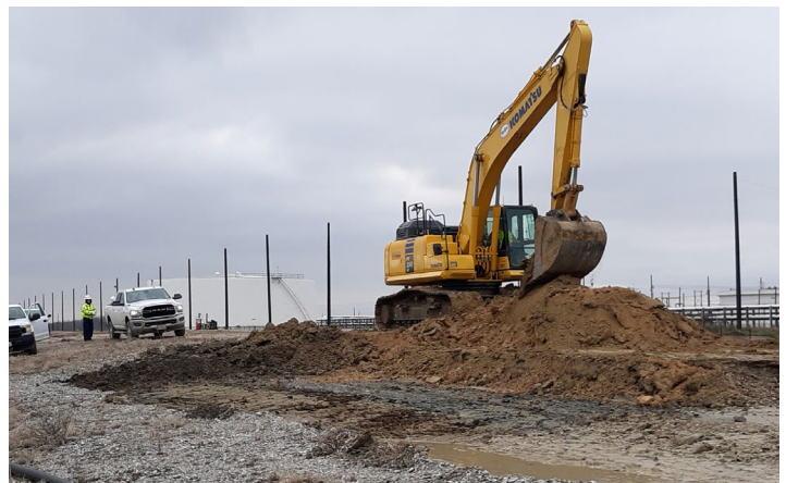
Construction on the S2G Port Arthur Project
