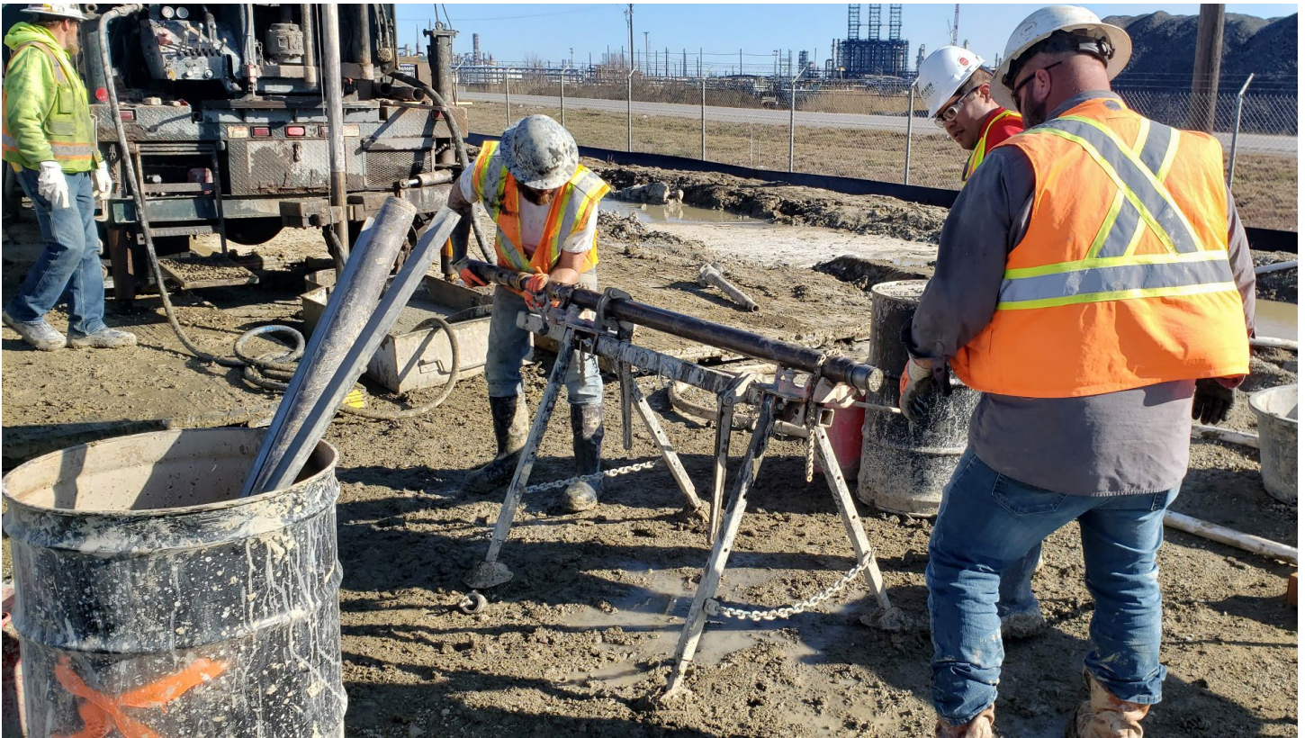
Contractors conducting geotechnical investigations on the Port Arthur Project
