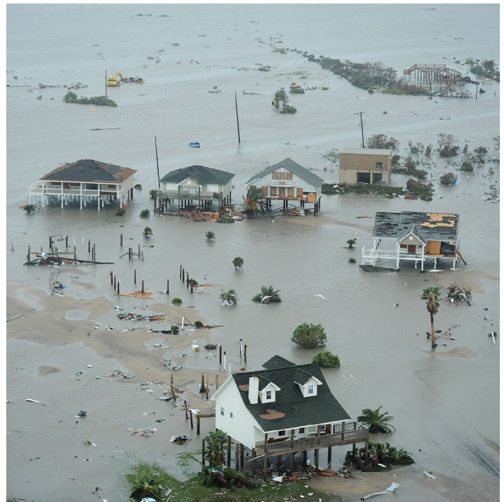
Galveston Island after Hurricane Ike
