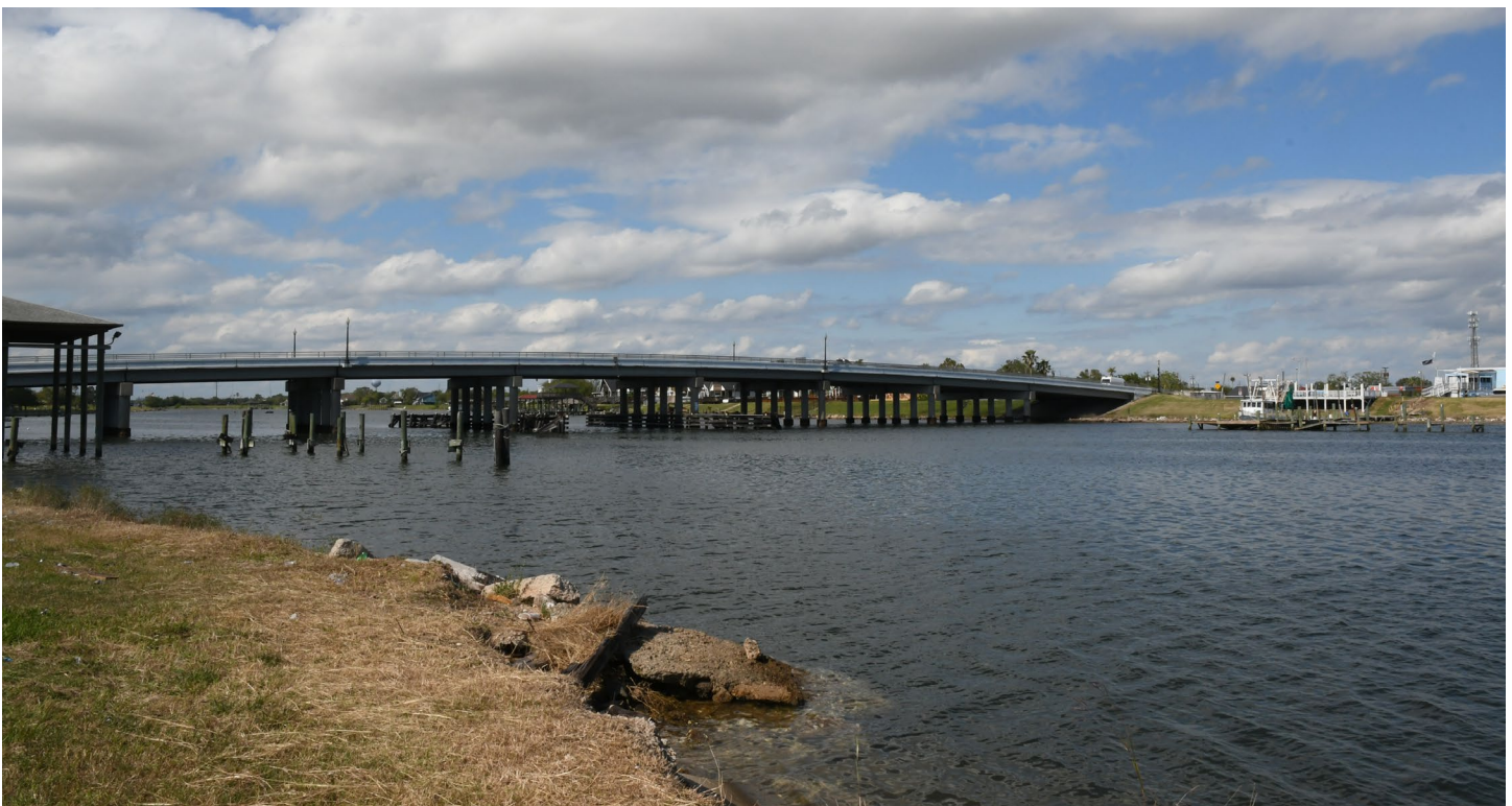
Velasco Boulevard Bridge in Freeport
